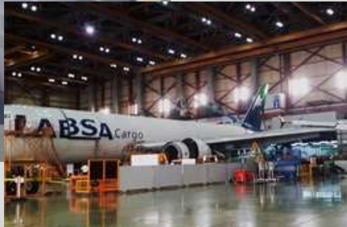
Hangar Lighting Installation Abu Dhabi_UAE
